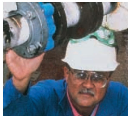
Gar-Seal Series 122L valve installed in monomer service.
